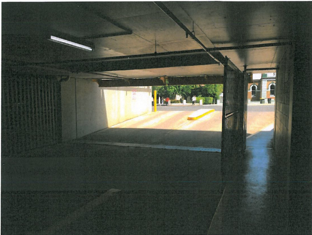
Plate 1: Existing car park entrance from Kite Street (note inward opening gates)
